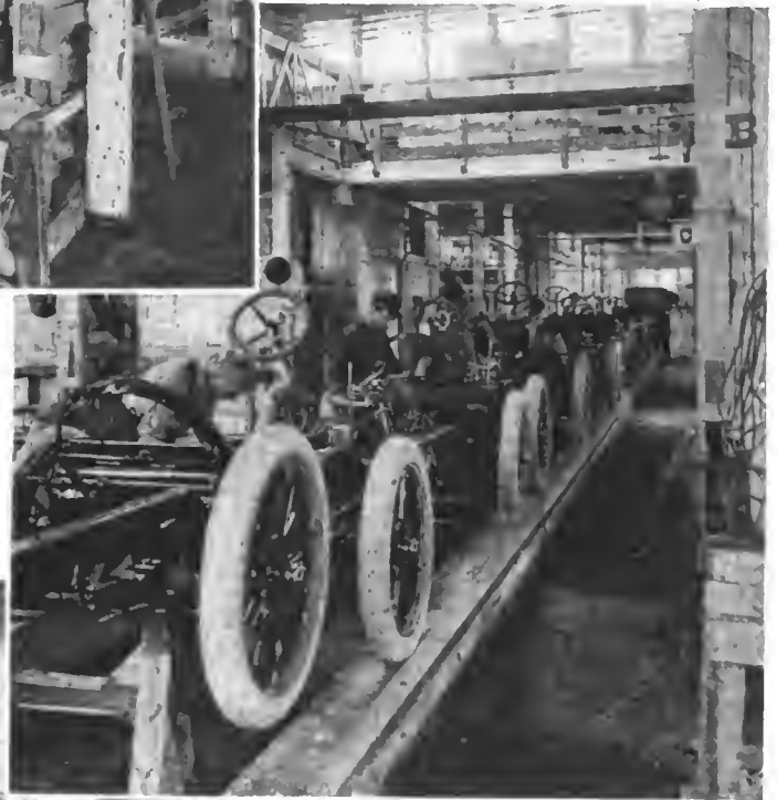
At the start of the assembly line in the factory of the Liberty Motor Car Co., Detroit, Mich. The chassis run down the track accumulating their component parts as they progress. Note the engine being lifted into place at the right and the overhead runways delivering wheels from the stockroom
